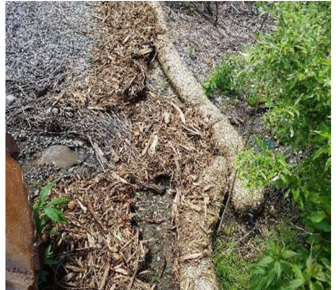
Fig 12: Straw wattle surrounding lay down yard off of Gosling Road needs to be staked in. Viewing west. (Jun 6, 2019).
