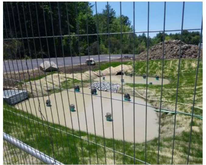
Fig 4: Rain garden along Colovos Rd. The rain garden is full of water. Viewing west. (Approx. 1330 on Jun 3, 2019).
