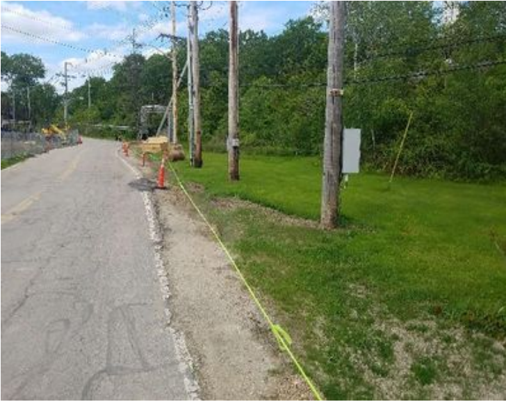
Fig 9: Proposed area east of Colovos Rd to discharge the trench water, with filter bag & BMPs installed. Viewing north. (Jun 5, 2019).
