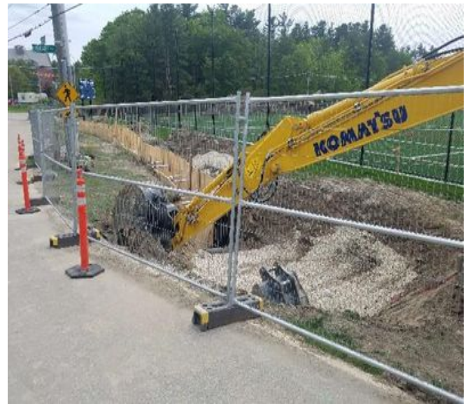
Fig 10: Repairs made and excavation filled with stone. Viewing south. (Jun 5, 2019).
