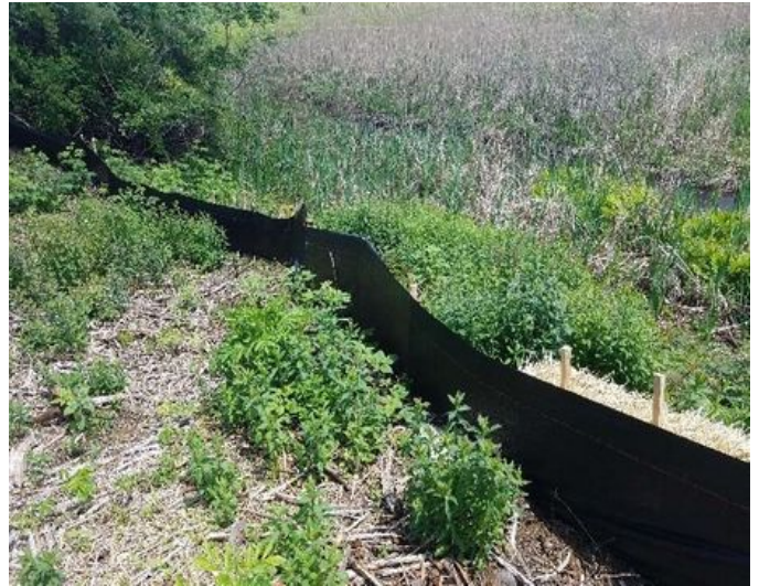
Fig 14: Silt fence near Str. F107-137 installed correctly. Viewing north. (Jun 6, 2019).
