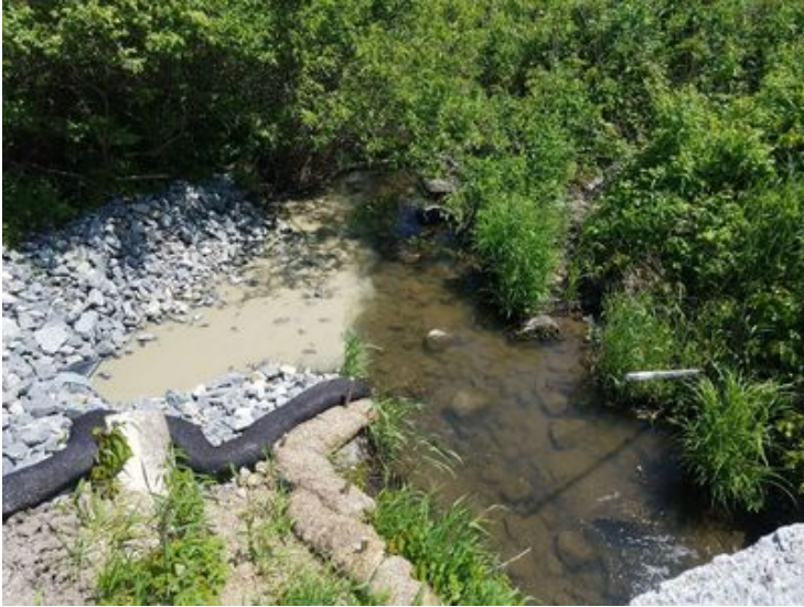
Fig 5: Discharge from the rain garden into College brook. Viewing east. (Approx. 1330 on Jun 3, 2019).
